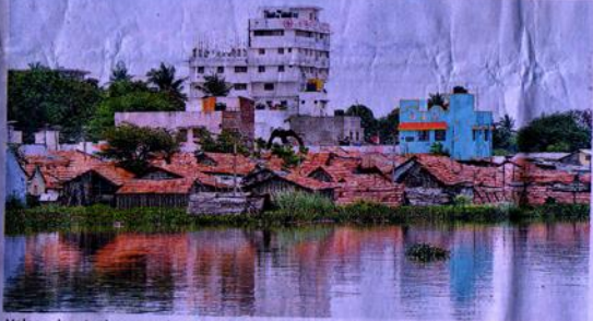
Valangulam tank encroached by huts. (Right) Singanallur tank in Coimbatore covered with hyacinth.
